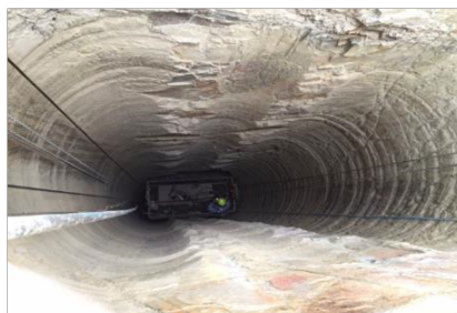
Figure 2: 27m deep shaft
