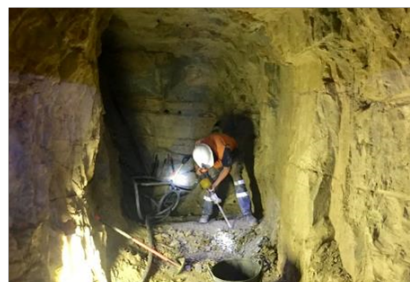
Figure 3: Miner drilling the drive at Goldsmith
